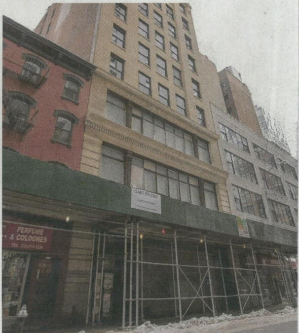
Pondicheri will occupy a ground-floor space at 15 W. 27 St.
